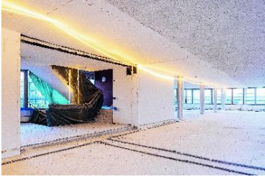
Image from Z2 during the renovation work
