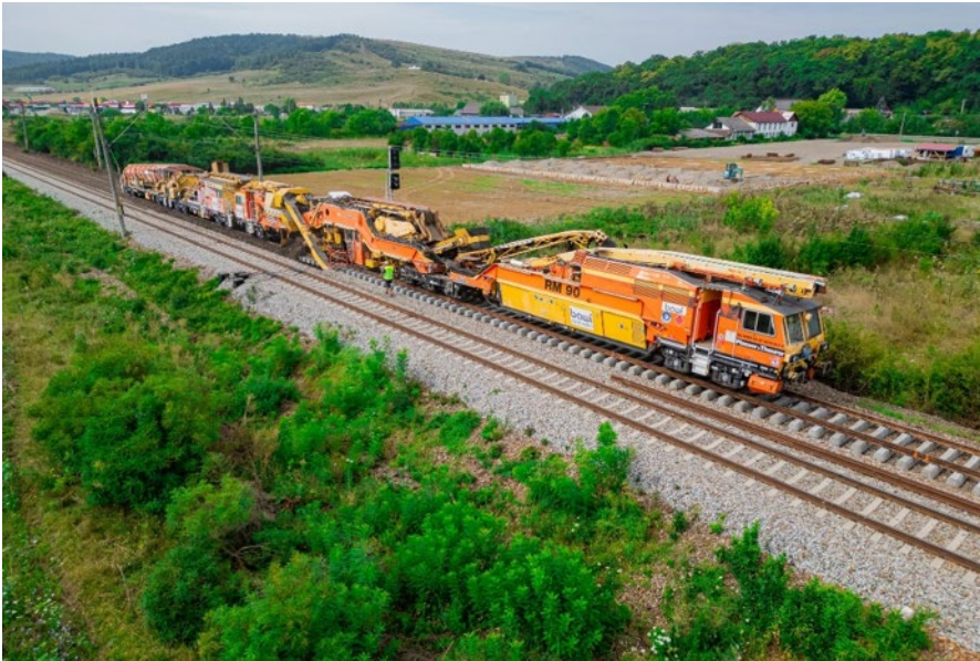
The Romanian railway construction specialist BAWI Construction is now part of the STRABAG Group. © BAWI construction
